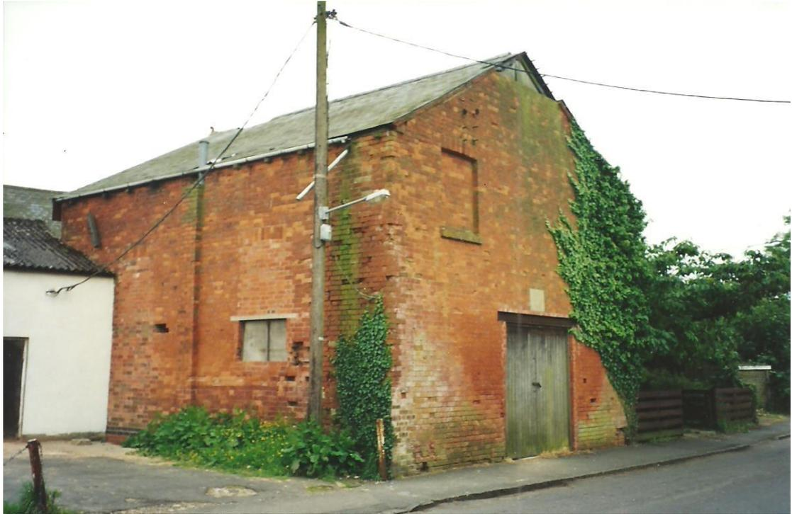
The Chapel was bought by an architect in 2005. While remaining true to the Chapel's original external appearance, the crumbling brickwork was replaced after the rear wall collapsed while new footings were being put in. An extension was built to the side on part of the adjacent factory site which the new owner acquired.
