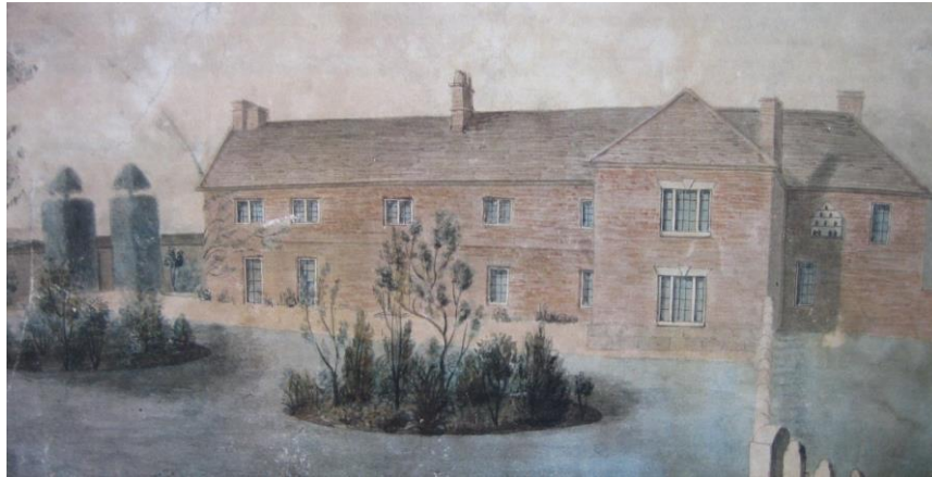
Barby Rectory south elevation c 1750
